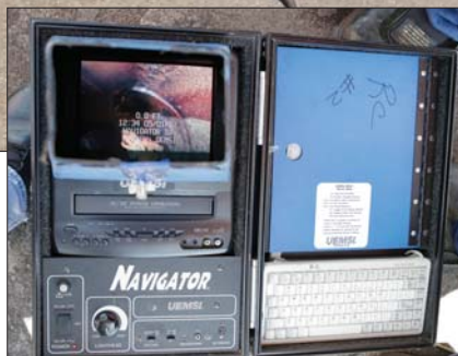
The light-colored object in the bottom center of the screen is a root that has entered a sewer line. RootX will be used to kill the root.
