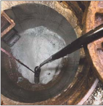
Top left: A map generated by Geomedia GIS software in the a city TV truck shows a neighborhood in which a crew is doing root control work using. Bottom left: A foaming pipeline root control formulation kills roots in the City of Fairfield's sewers. Right: Assistant foreman Jason Turner controls a remote camera as he views live video of sewer lines from the TV truck.
