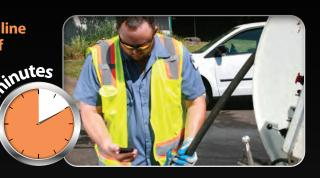
After 10 minutes or the extended amount of time for heavier grease buildup, turn the jetter back on high and begin jetting. Retrieve the nozzle back at a slower rate than you went up the line allowing the high pressure of the spinning nozzle to emulsify and remove the grease. Hose retrieval rates should be between the 1 to 3 feet per second.
