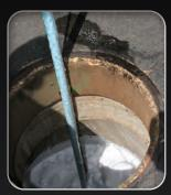
Once the jetter nozzle is back to the downstream manhole, shut of the water and remove the jetter hose from the line and proceed to the next section of pipe to be treated. If you need to refill the tank with water and Grease-X° Jet before the next application do so at this time. Grease-X° Jet should be applied as needed to maintain the line and restore pipe flow capacity.
