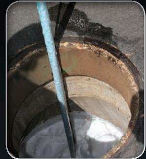
**6** Once the jetter nozzle is back to the downstream manhole, shut off the water and remove the jetter hose from the line and proceed to the next section of pipe to be treated. If you need to refill the tank with water and Grease-X® Jet before the next application do so at this time. Grease-X® Jet should be applied as needed to maintain the line and restore pipe flow capacity.
