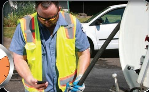
**5** After 10 minutes or the extended amount of time for heavier grease build-up, turn the jetter back on high and begin jetting. Retrieve the nozzle back at a slower rate than you went up the line allowing the high pressure of the spinning nozzle to emulsify and remove the grease. Hose retrieval rates should be between the 1 to 3 feet per second.
