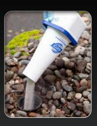
Add 38 litres of water per 908g of product use into the cleanout to push the foam down throughout the sewer line.
