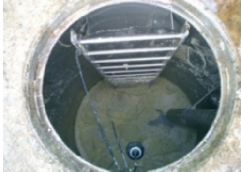
Grease build-up in wet well before GREASE-X GT® treatment
